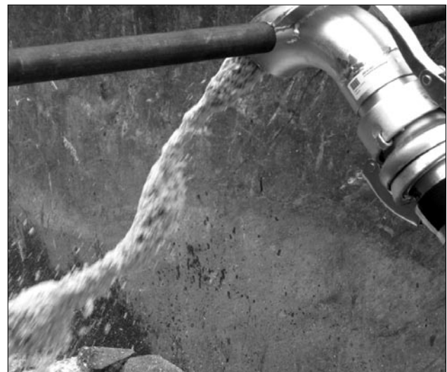
Fig. 5: Discharge of VIB 25 E-SY castable into the collecting container
